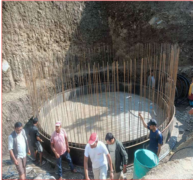
100 cum RCC Tank Aathbikot-9
